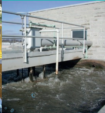
Aeroductor Aerated Grit Removal System
