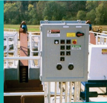
In-Line Grit Collector Grit Removal System
