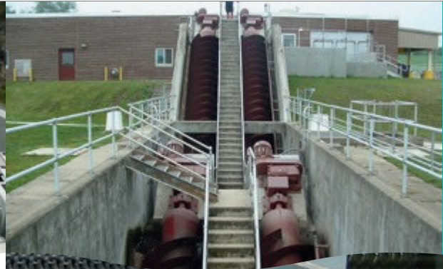
Open Screw Pump – Dual Stage Design
