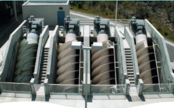
Open Screw Pump – Single Stage Design
