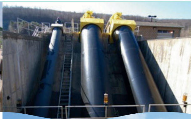
Type “C” Enclosed Screw Pump
