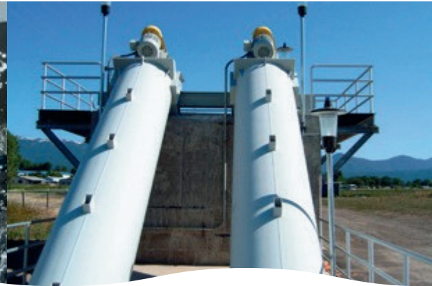
Type "S" Screw Pump Tube Vents
