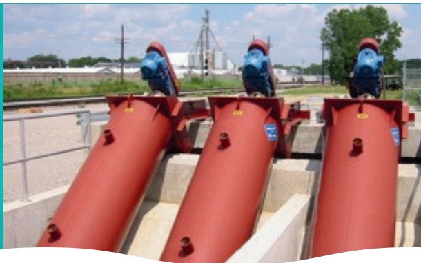
Type “S” Enclosed Screw Pump
