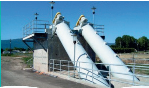
Type "S" Enclosed Screw Pumps
